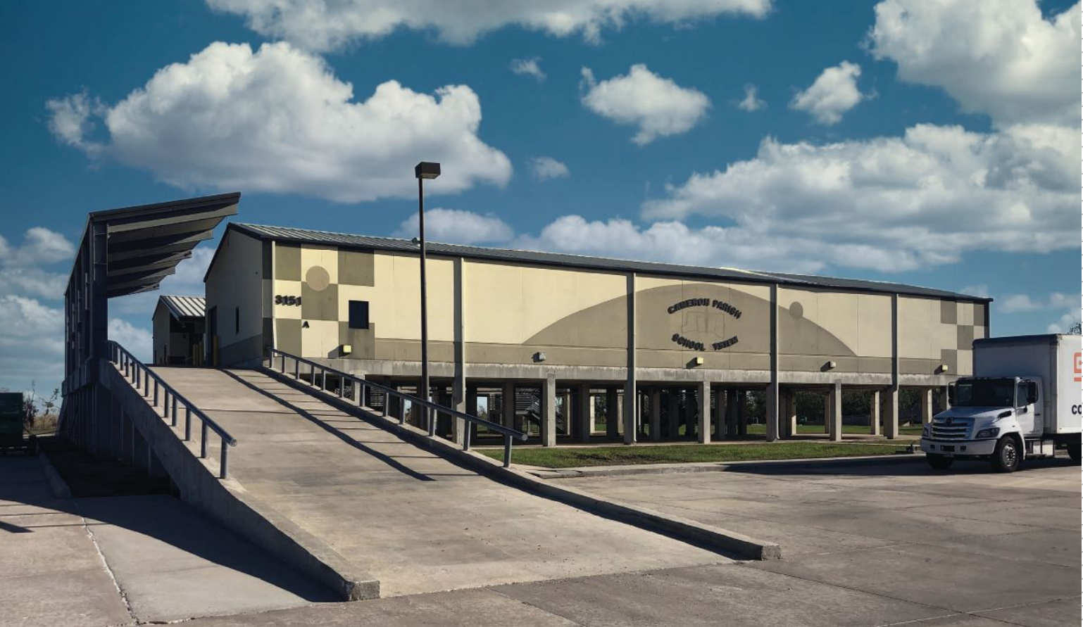
Used to store perishable food and dry goods for school cafeterias in Cameron Parish, this warehouse was elevated to minimize the risk of flooding from storm surge. All photos: Jessica Wene Photography.
